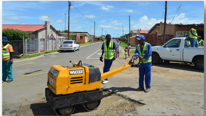
Street Patching in Mlangeni
