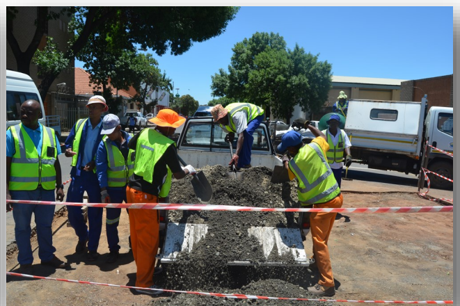
Street patching as part of service delivery
