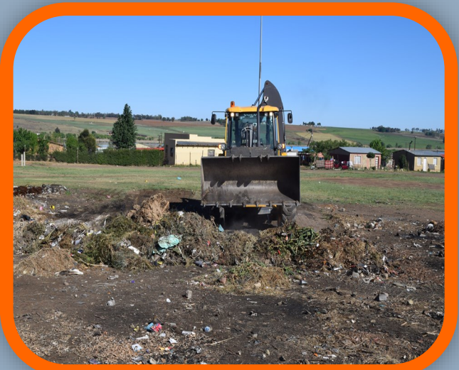
Cleaning of corner dumps
